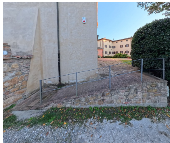
6 Church side ramp
